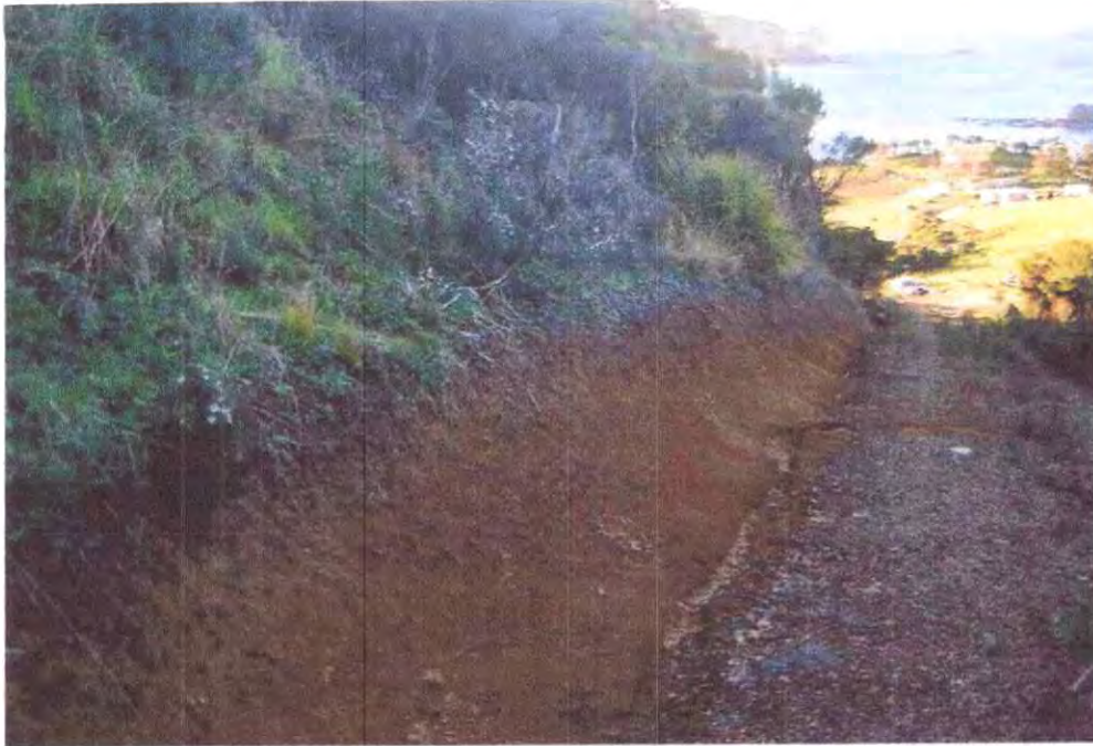
Plate 1: View North along existing road showing 100 Metre long soil exposure
